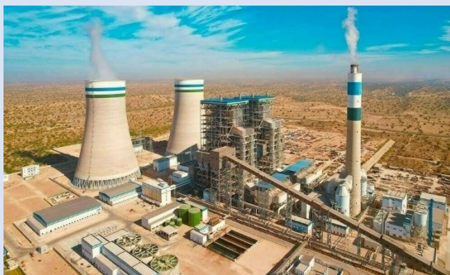
Jamshoro Coal Power Project (Pakistan)
